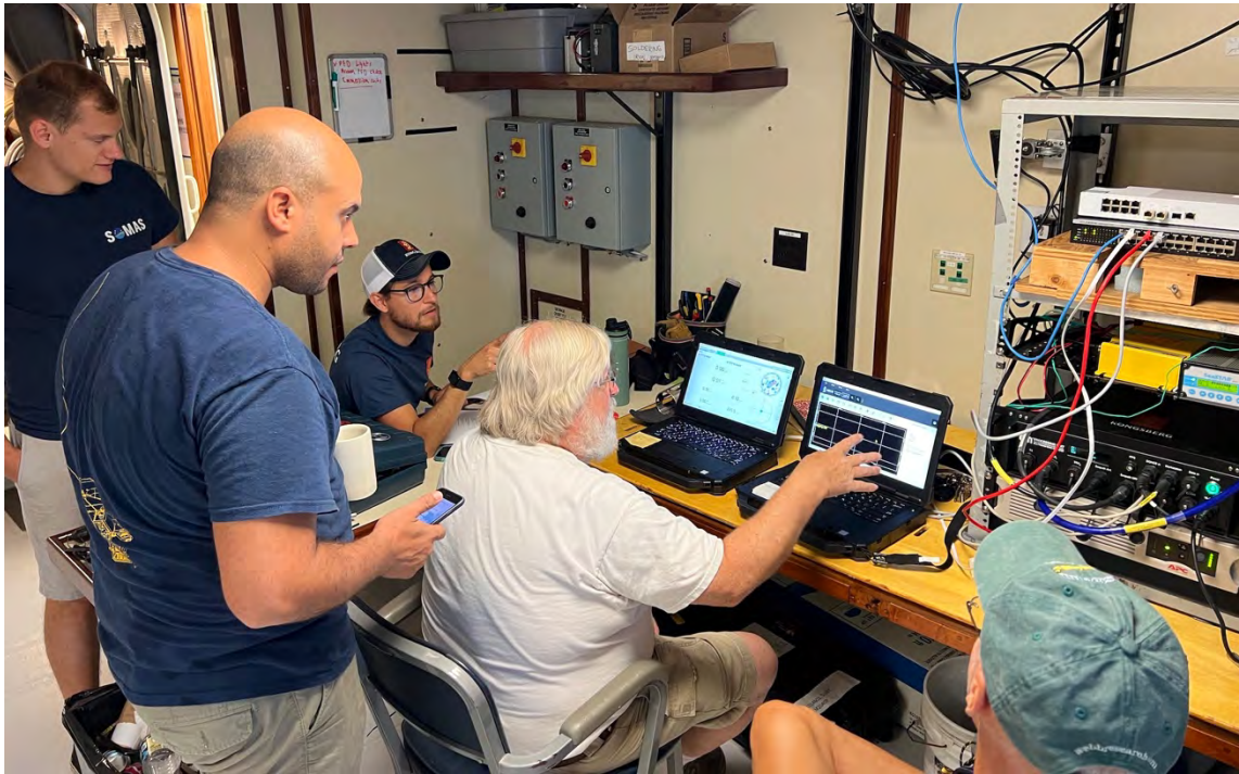
Figure 2-3 Installing the data acquisition system in the dry lab (from left to right - Jason, SBU graduate student; Mohammed, SBU Post-doc; Dan, Kongsberg technician; Roger, Chief Scientist; Dennis, UConn/LISMaRC technician).
